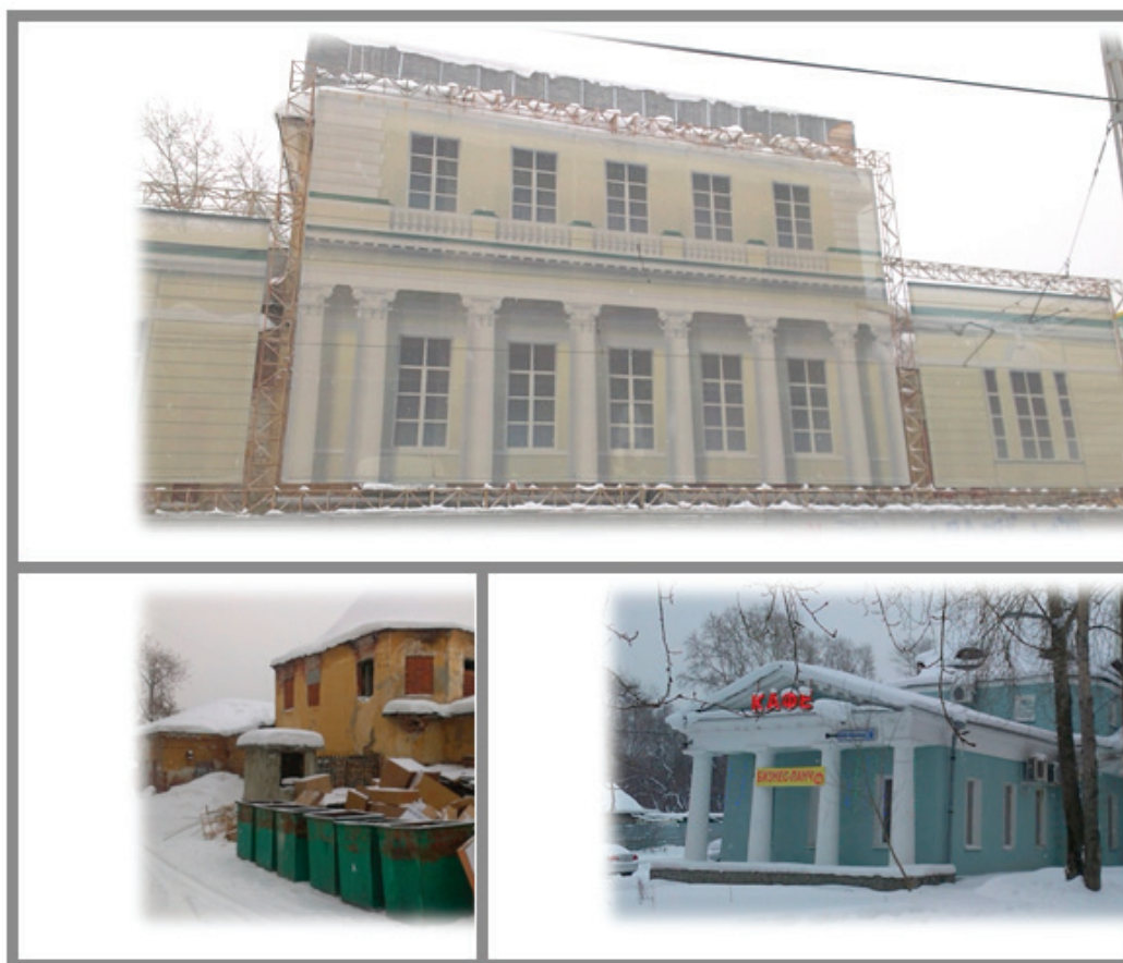
Figure 6. Photos of present condition of the hospital
