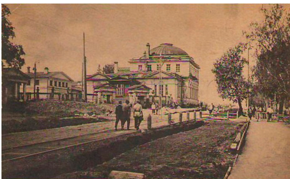
Figure 5. The hospital building after reconstruction without 8-columned portico. Source: www.mugiso.midural.ru/region/okn/estateekt.php?ELEMENT_ID=733
