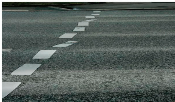
Fig. 1. Deformations of wheel tracks formed on pavements as a result of vehicle movement
