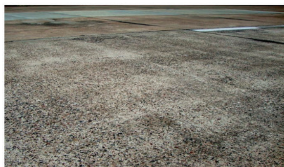
Fig. 2. Disruptions (depth) and cracks caused by deformations in the base layers of the road surface
