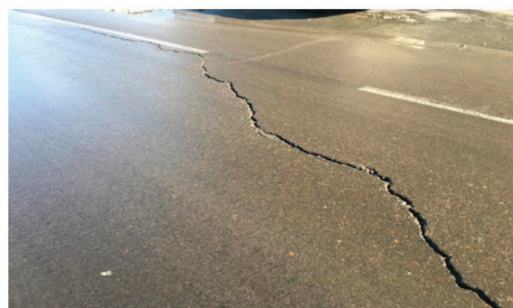
Fig. 2. Disruptions (depth) and cracks caused by deformations in the base layers of the road surface
