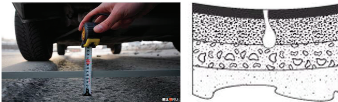
Fig. 1. Wheel track deformation in asphalt concrete pavement
